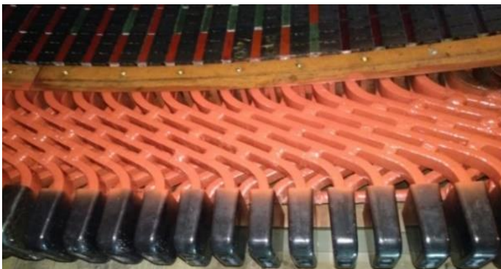
Figure 11. Lower Overhang Area after Repairs
